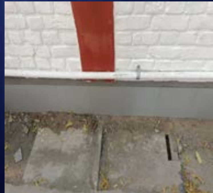
Skirting tile work on boundary wall
